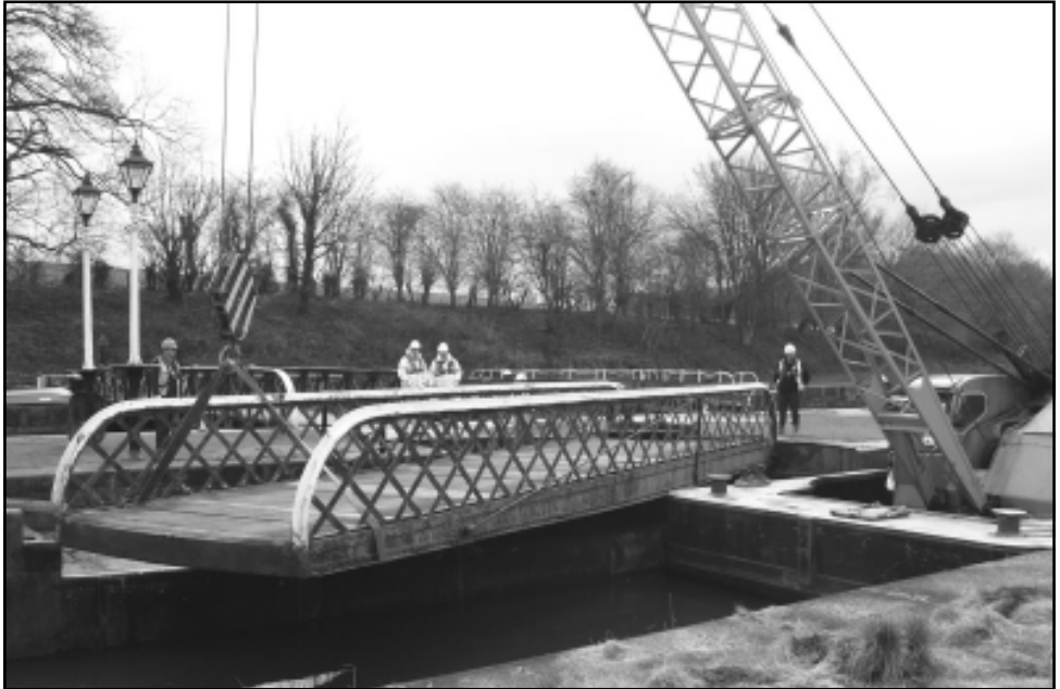
The bridge was opened whilst being supported by a floating crane
