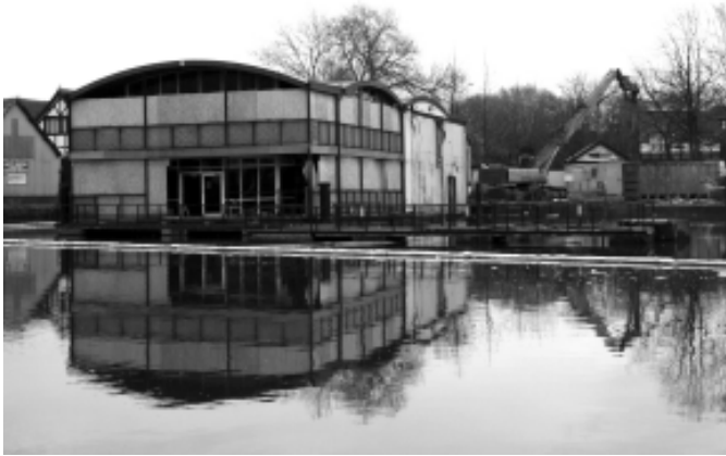
Demolition underway in November 2009
